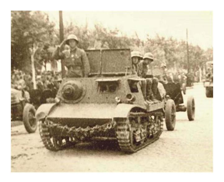
The T-20 Komsomolets Artillery Tractor was primarily used for towing light artillery pieces. Its tracked design enabled it to traverse rough terrains, ensuring that artillery units could be rapidly deployed. This vehicle played a significant role in the Red Army's artillery operations.
