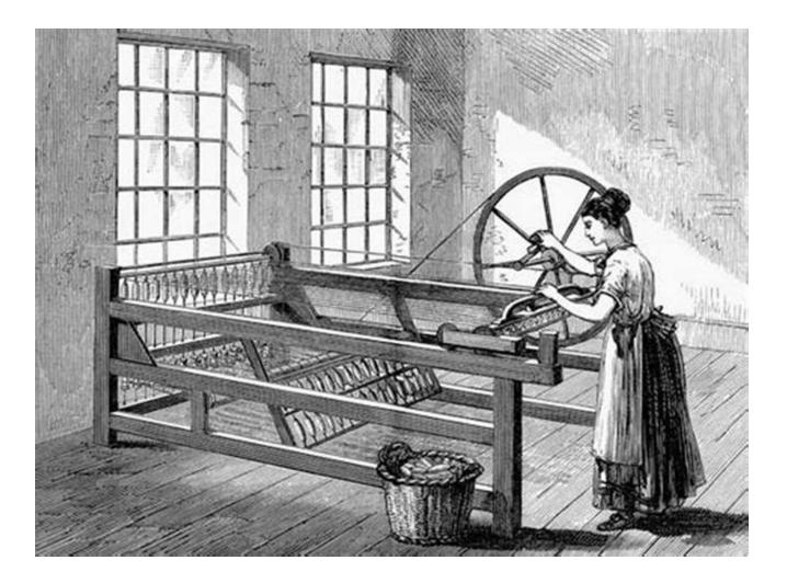
One of the key inventions during the Industrial Revolution was the Spinning Jenny, a multi-spindle spinning frame. Patented by James Hargreaves in 1764, this device revolutionized the textile industry by allowing a single operator to spin multiple threads simultaneously. The Spinning Jenny increased production efficiency and played a vital role in accelerating the growth of the cotton industry.
