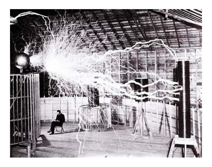
At the heart of Tesla's experiments was his revolutionary invention – the Tesla coil. This high-voltage transformer allowed Tesla to generate and control extremely high-potential and high-frequency alternating currents. It became the cornerstone of his inventive endeavors and showcased the immense possibilities of AC electricity.
